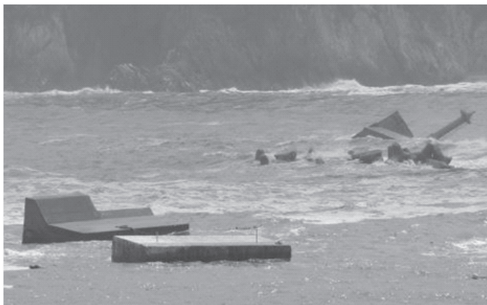
Fig. 6. A variety of concrete debris from breakwater and seawalls offshore of Tarō which observed during the 2011 EEFIT mission [3].
