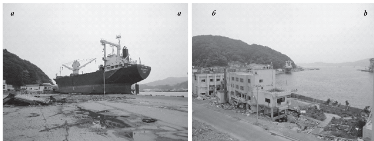
Fig. 4. A cargo ship dumped to a pier in the Kamaishi Port, Japan (a) and the scour around concrete building in Kamaishi by the Great East Japan Earthquake and Tsunami (b) (photos by Ahmet Cevdet Yalciner).
